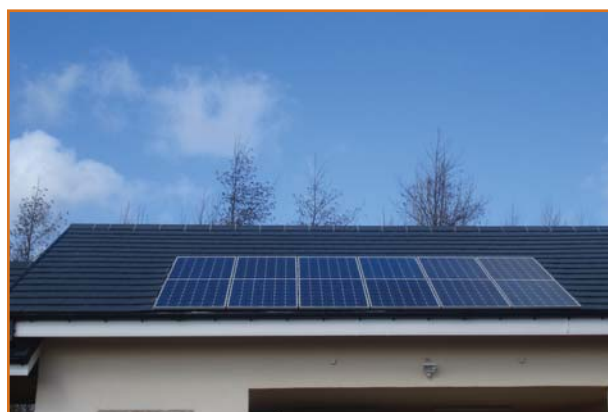
1.98kWp CareyGlass Solar grid connected system on a passive house in Newbridge
