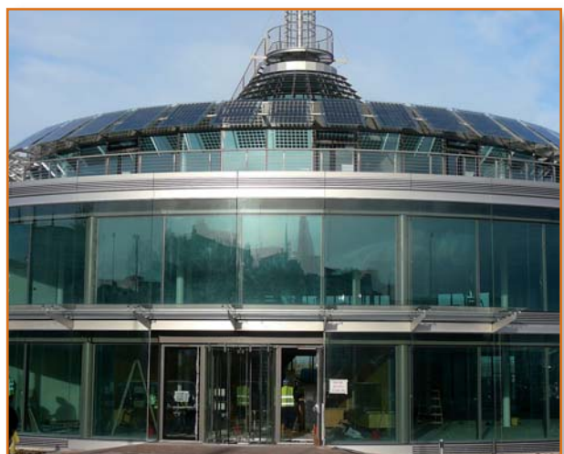
Commissioner for Irish Lights Headquarters in Dun Laoighre which uses 32 PV modules & 2 inverters to generate solar electricity
