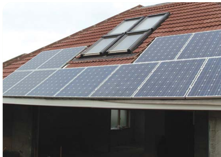
1.98kWp grid connected PV system in Mount Merion, Dublin'
