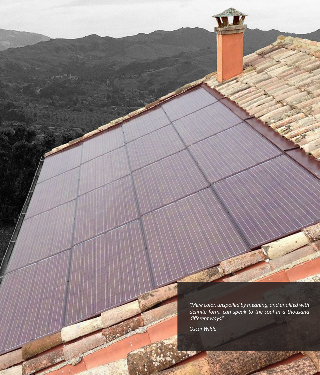
Detail of special BIPV (Solrif®) frame
